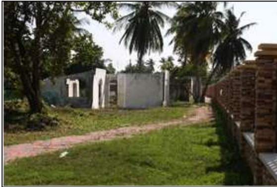
Figure 1: Remnants of tsunami-damaged houses in the study area (Source: Field Observation)
