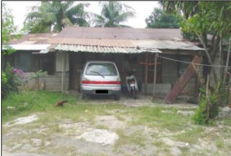
Figure 1: An example of structural adaptation depicting a house with concrete lower wall. (Source: Field survey)
